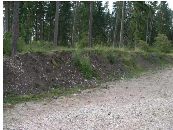
Figure 2-10: Bank at Grafenwöhr Training Area. They were situated next to roads and mostly consisted of a gravelled core, covered with soil. They are used for tactical training and to protect from lime dust.
