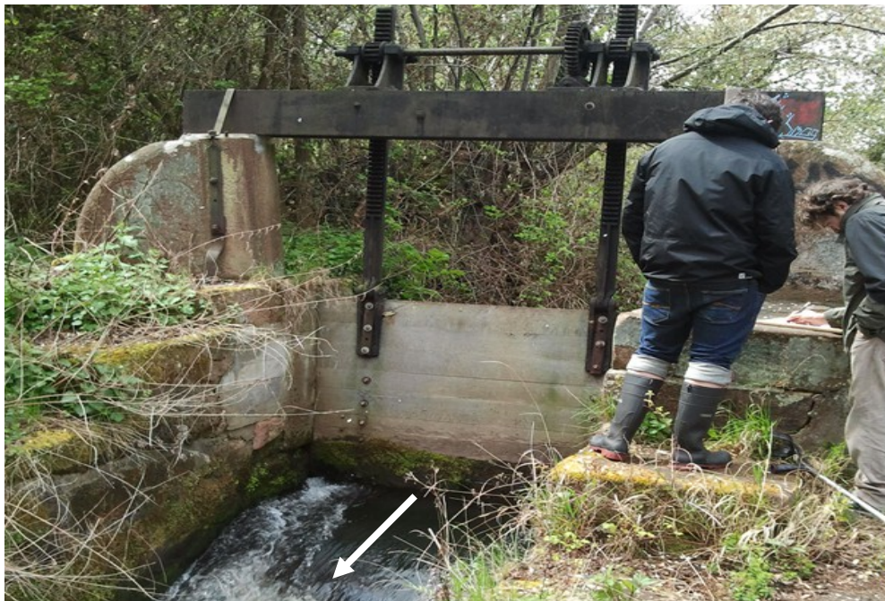
Figure 1-2: Example of a small in-stream dam that impounded one of the studied streams. The white arrow shows the direction of water movement.
