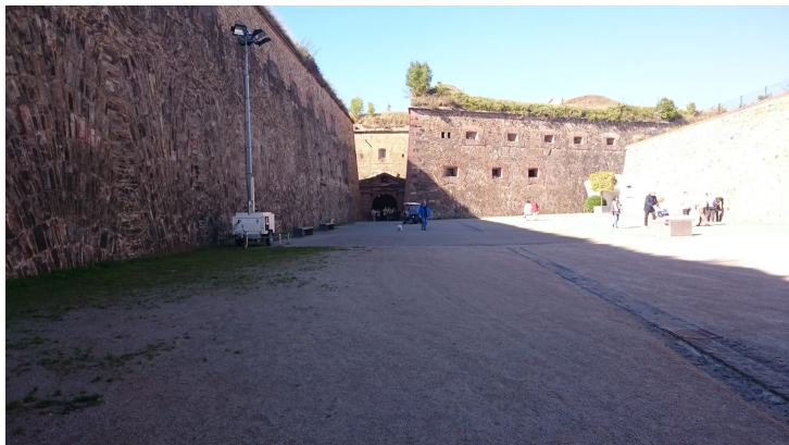
Figure A.29: Spatial: width of path to tunnel
