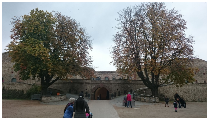
Figure A.22: Spatial: height of tree in front of tunnel
