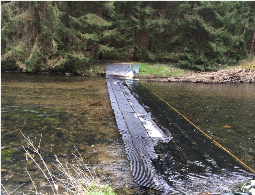
Figure A.3: Dynamic fish weir during mid-flow conditions. Picture taken on March 23, 2016. The discharge at the gauge Heimborn approximately 4 km upstream of the experimental site was 2.2 \text{ m}^3\text{s}^{-1} around the time the photograph was taken.
