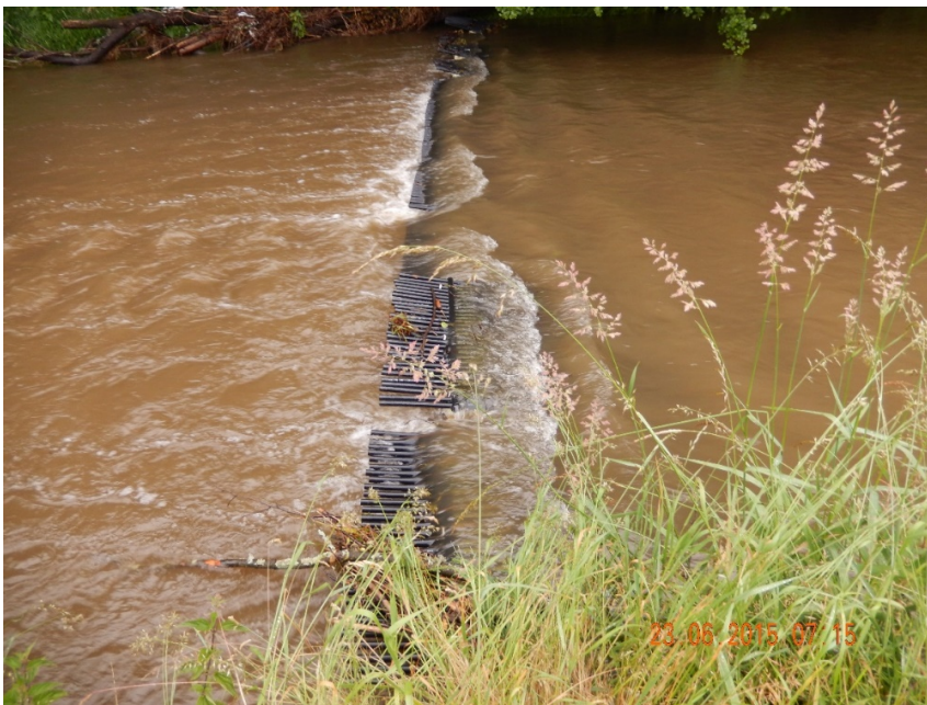
Figure A.4: Partly submerged dynamic fish weir during high-flow conditions. Picture taken on June 23, 2015. The discharge at the gauge Heimborn was 4.1 \text{ m}^3\text{s}^{-1} around the time the photograph was taken.
